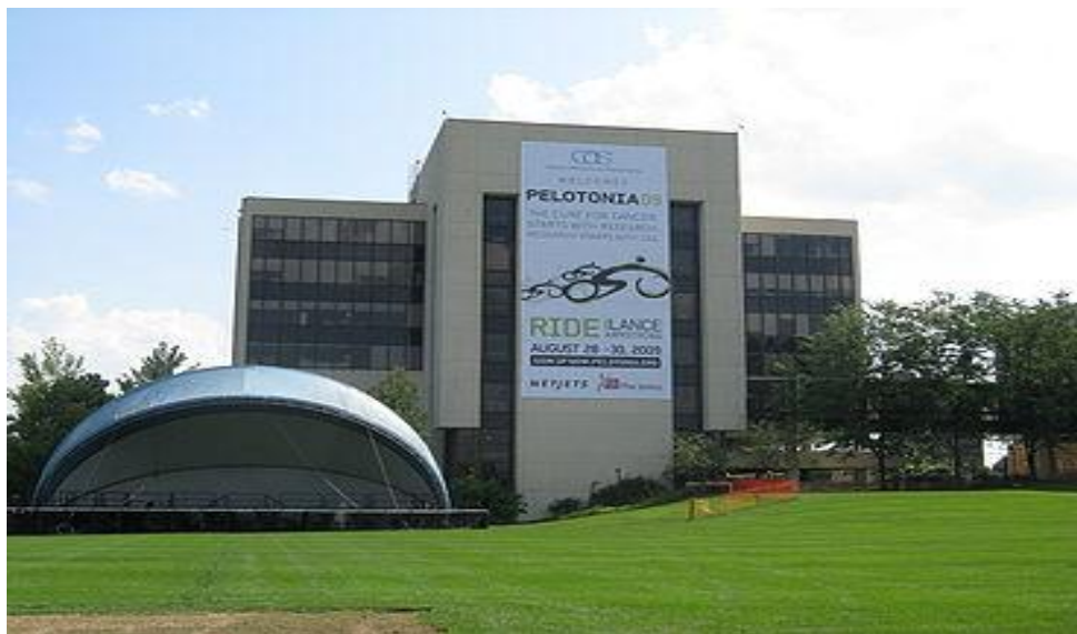
Figure 4: Chemical Abstracts Service Building B in August 2009. Columbus, Ohio.
